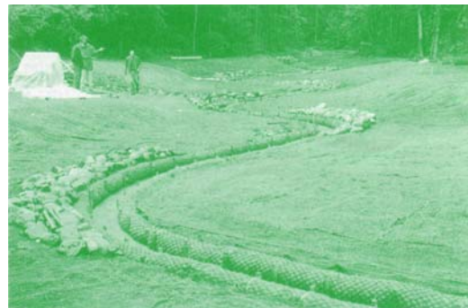
A shallow stream bed under construction in Blue Heron Park will reduce flooding and erosion, much as the daylight wetlands will in the Olympic rowing proposal.
